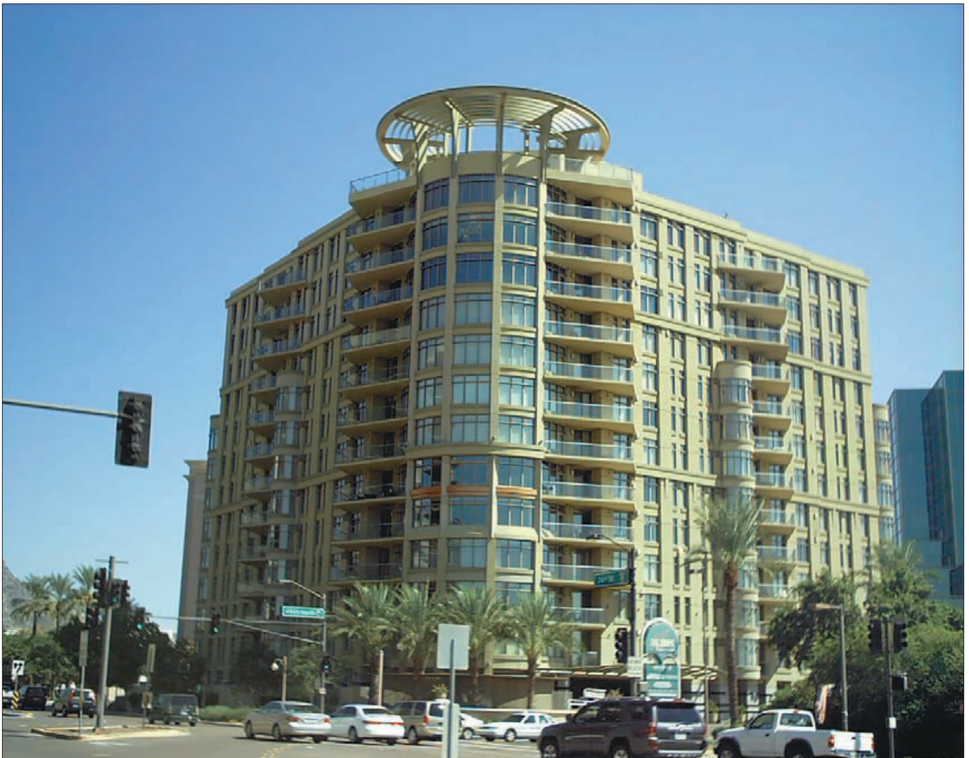
Esplanade Place is using submeters to monitor and allocate common area costs and provide monthly tenant billing statements, in addition to identifying previously hidden energy savings opportunities.
